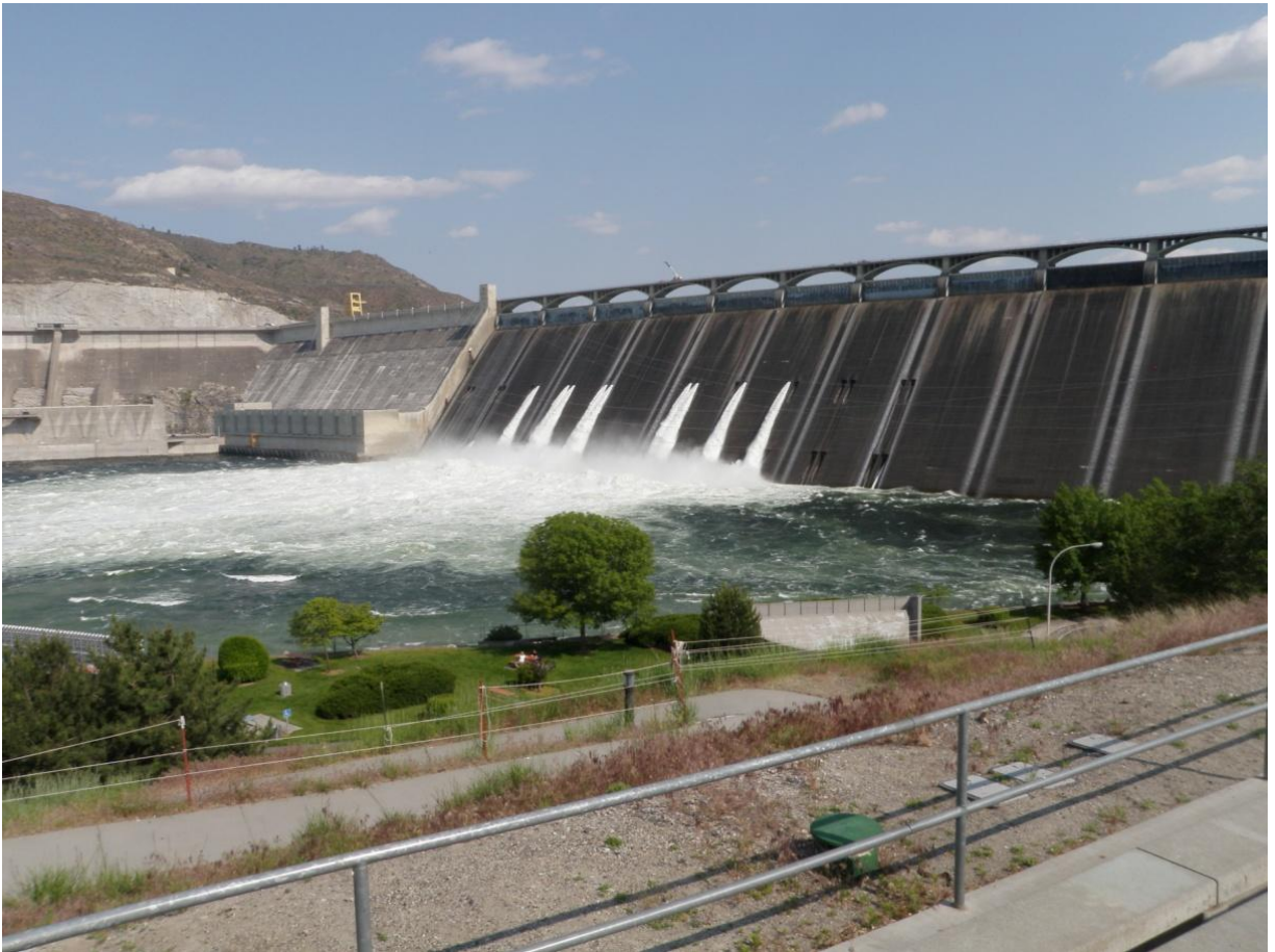
Figure 2 - Downstream view of Grand Coulee Dam showing the third power plant on the left and 40 river outlets on the face of original dam below the spillway crest.
