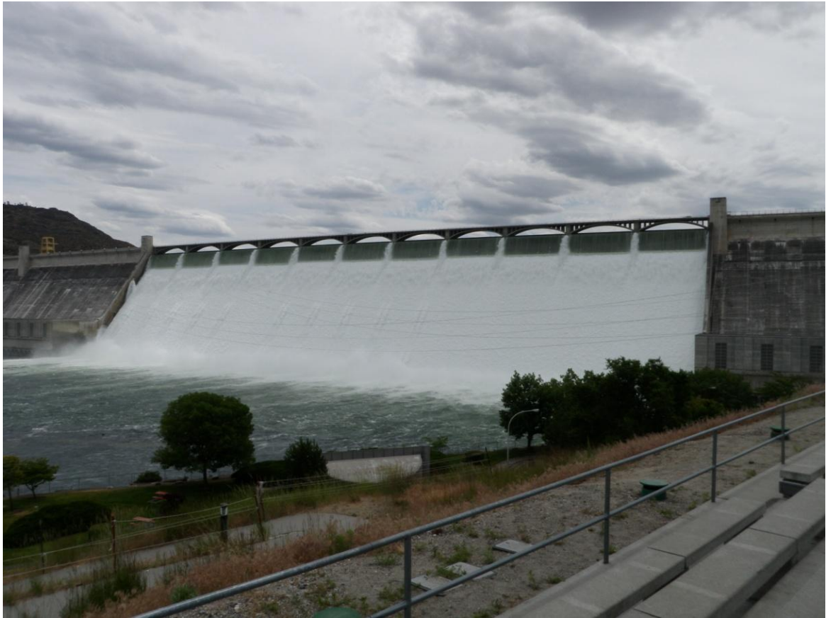
Figure 3 - Grand Coulee Dam spilling, July 2011.
